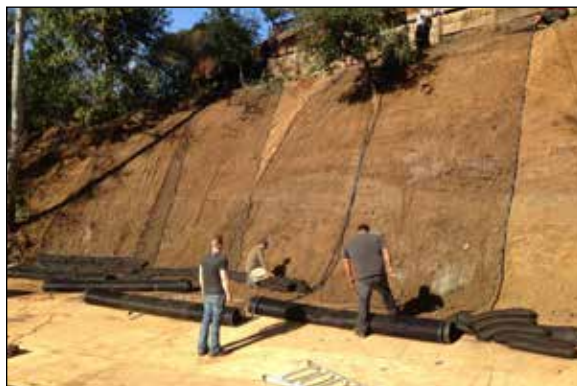
Project site, GreenLoxx VSF Installation
