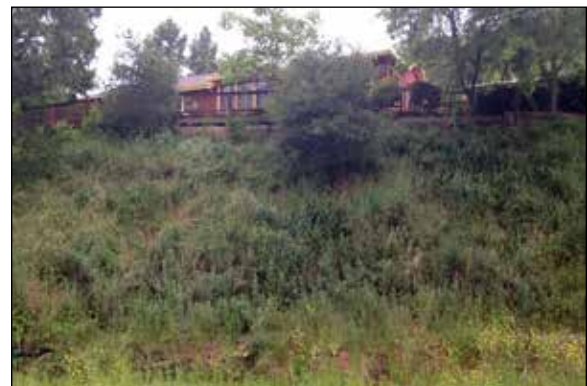
GreenLoxx VSF, after
