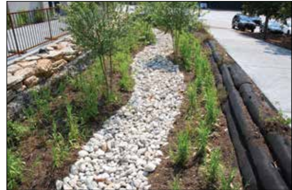
Bioswale installation in urban application.
