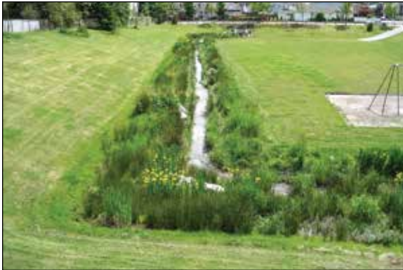
Bioswale installation in residential application.
