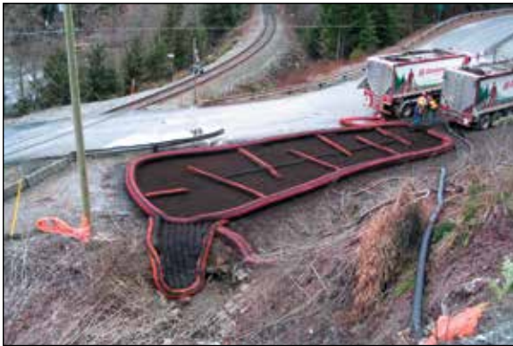
Filtration system installation
