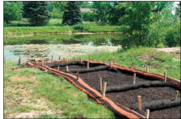
Filtration "cell" system installation
