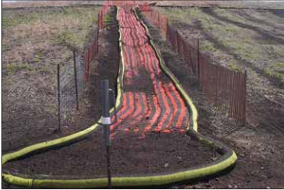
Installation of channel protection
