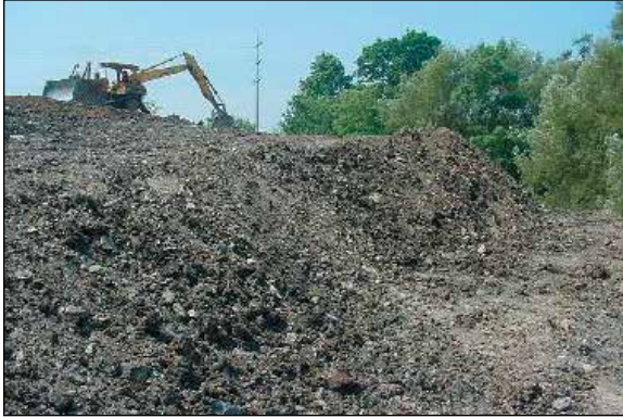
Industrial Site Remediation
