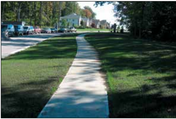
Compost Vegetated Cover is generally used for rapid vegetation establishment.
