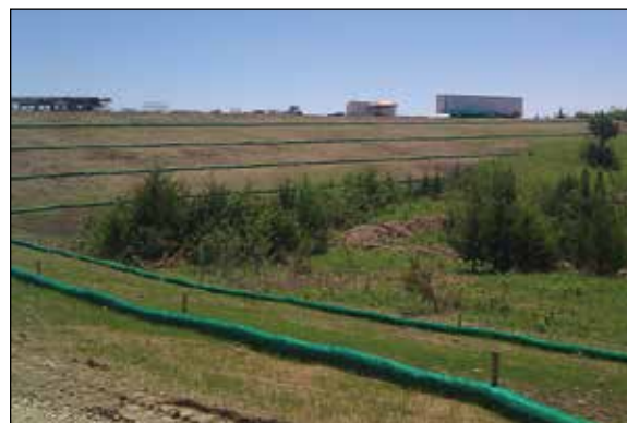
Aid vegetation establishment by reducing soil erosion
