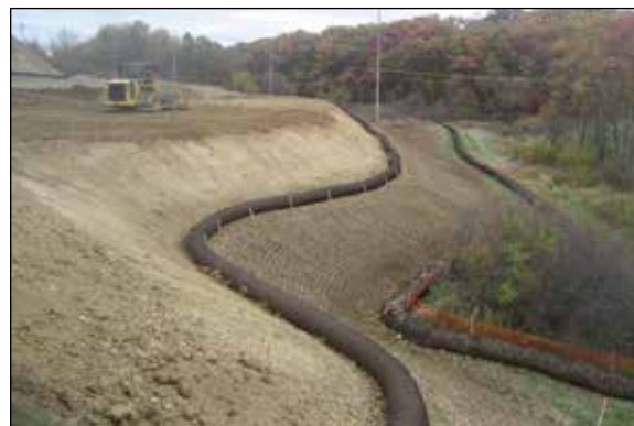
Minimize erosion of bare soils by runoff velocity reduction
