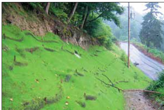
Vegetated Slope Interruption for permanent option
