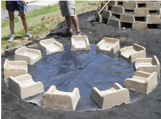
Figure 1a. Each green wall is designed with an underlying impervious base layer (Foreground). Blocks are arranged in 5 staggered tiers (Background).
