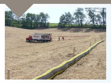
The mesh you choose matters. Filtrexx Blower Truck Mesh is the original compost sock mesh for field installation with blower trucks or track machines.
