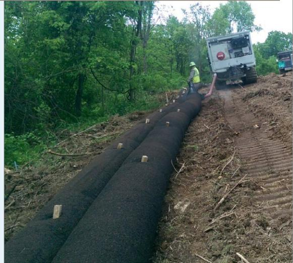
The mesh you choose matters. Filtrex Blower Truck Mesh is the original compost sock mesh for field installation with blower trucks or track machines.
