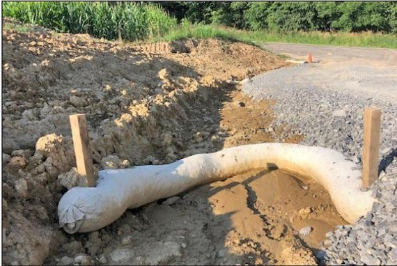
Filtrexx SiltSoxx NATURAL PLUS+ used as Check Dam.
