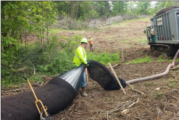
BASIC PLUS+ Blower Truck Mesh field installation.
