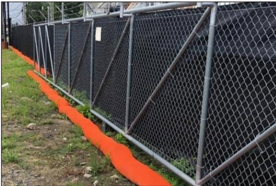
Filtrexx SiltSoxx EXTREME used in rugged conditions.
