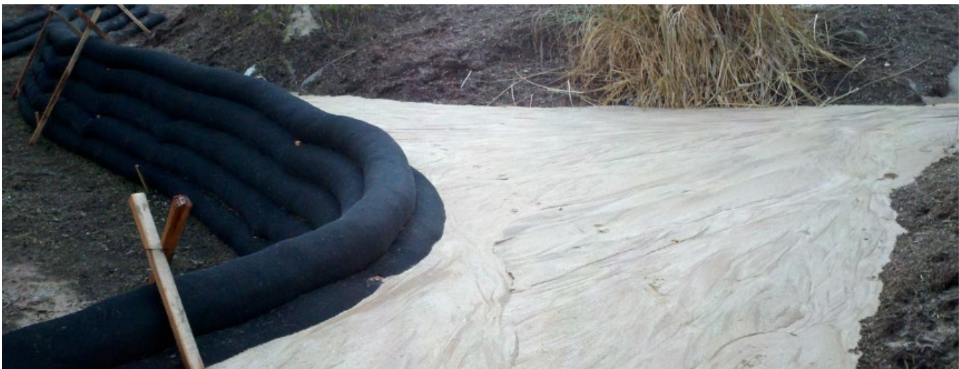
Sediment trap, 12-inch diameter filter socks in pyramid stack, photo courtesy of Filtrexx
