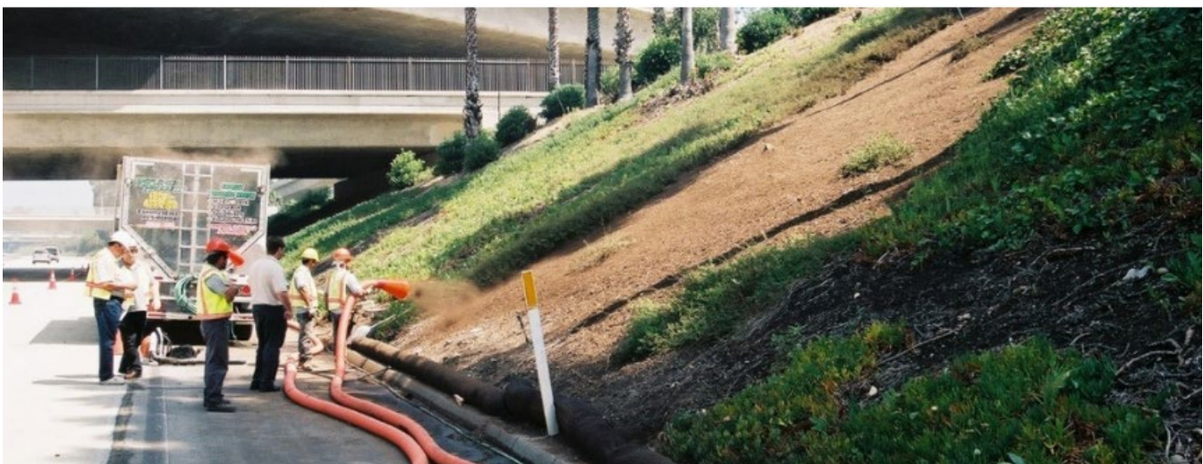
Roadside application of compost blanket, photo courtesy of Caltrans
