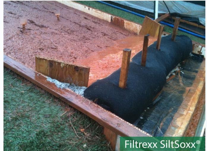
The performance difference between compost filter socks that adhere to federal and state specifications for mesh and media versus those that do not meet these specifications is quite substantial.
