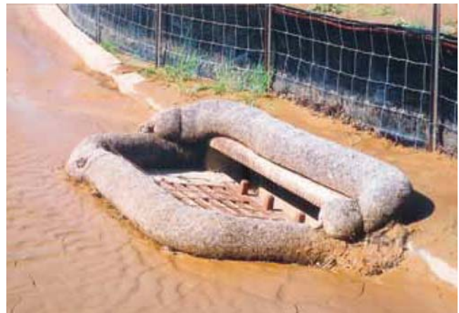
Figure 4 Compost filter sock curb inlet
