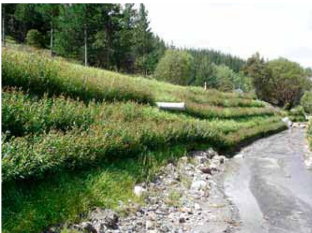
Figure 6 Vegetated compost filter socks
