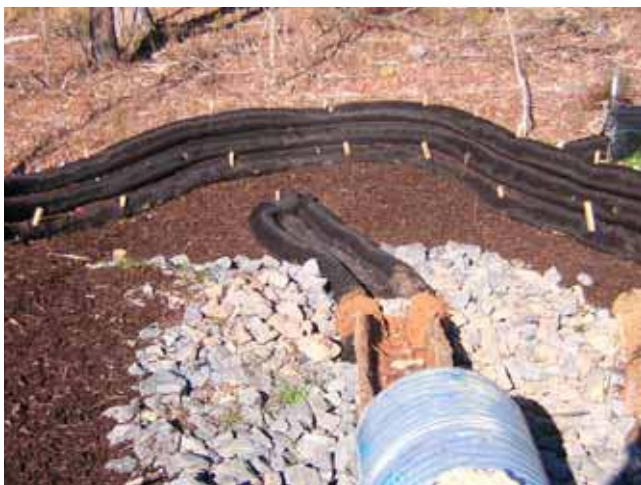
Figure 2 Compost filter socks used for capturing sediment
