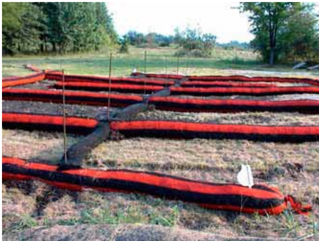
Figure 5 Compost filter sock biofiltration system
