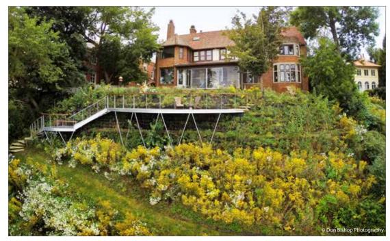
The living wall consisted of lightweight geo-foam block backfill material, soil anchors, and 3" galvanized pipe tied to layers of geogrid wrapped around every two layers of the GroSoxx® at the face of the wall. A native plant and seed mix was created specifically for the cultural needs and stabilization properties of the plants on the site.
