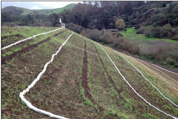
Filtrexx SiltSoxx NATURAL ORIGINAL used as Slope Interruption.
