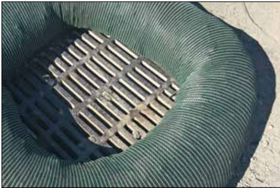
EnviroSoxx used around a drain/inlet.
