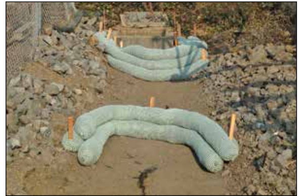
EnviroSoxx used as check dam.
